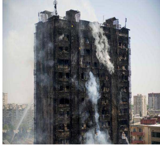
Resim 2. Grenfeel Tower Fire [2]
